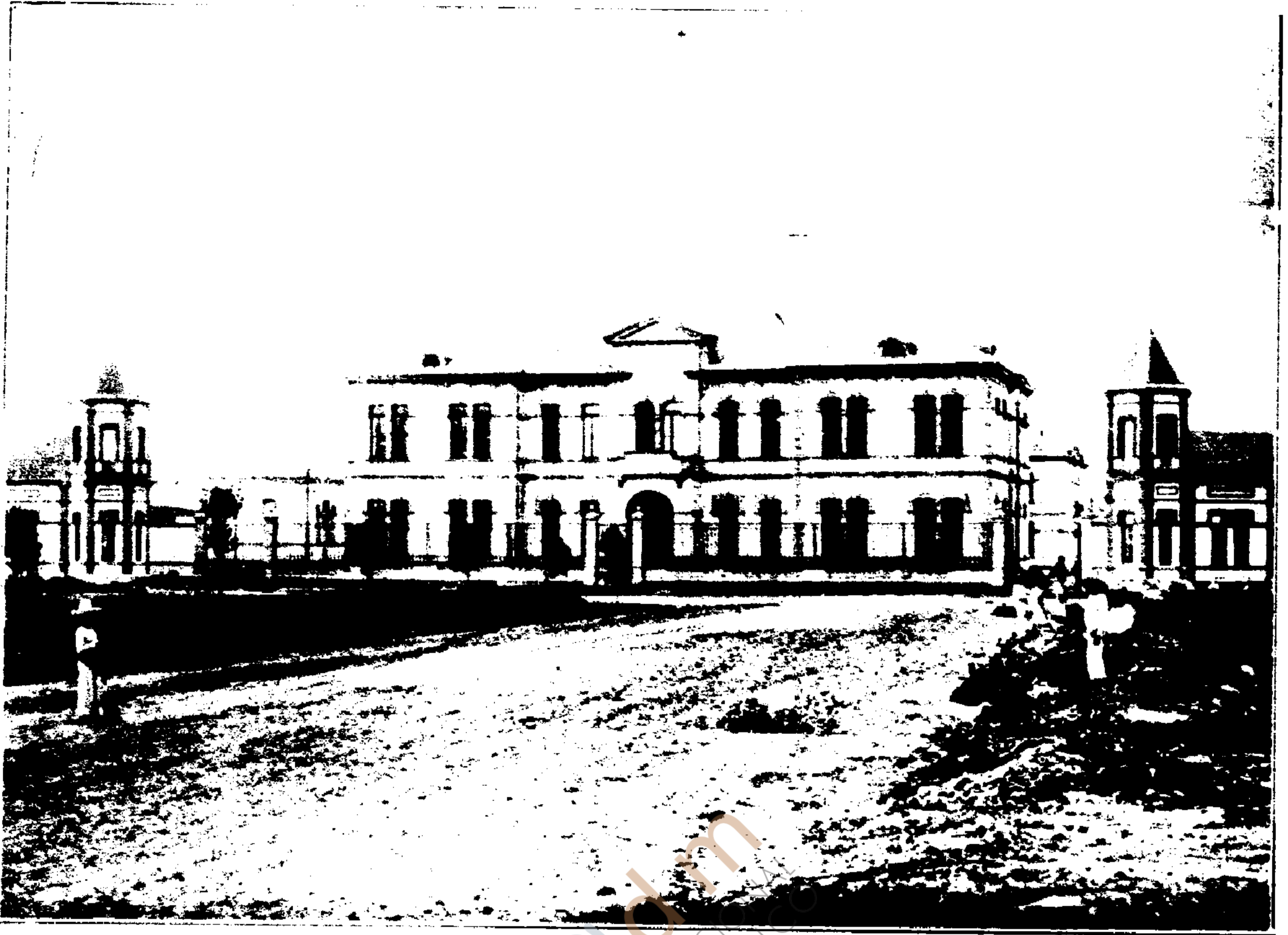
HOSPITAL GENERAL - CALLEADA PRINCIPAL
